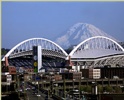
Seahawks Stadium & Convention Center Civil Design by George Franklet, PE ACM Engineering Principal Engineer
